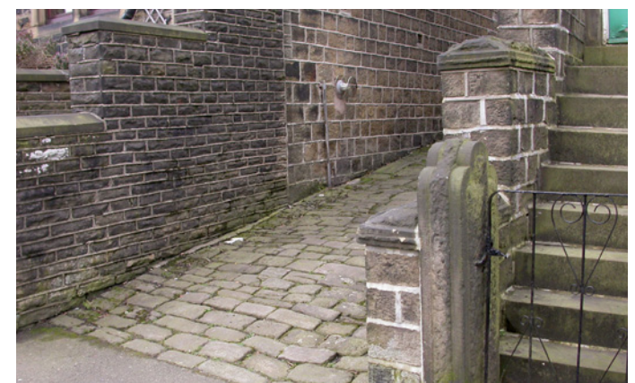
Setts, walls and gateposts in Marsden
